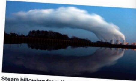
Steam billowing from the cooling towers of Vattenfall's Jaenschwalde brown coal power station is reflected in the water of a lake near Cottbus, eastern Germany December 2, 2009.
